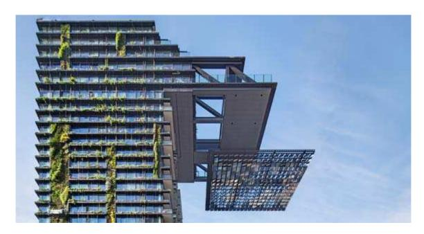
The Sydney high-rise also features Nouvel's signature giant cantilever. Extending from level 29 of the taller east tower, it supports a 'sky garden' above and a spectacular mirrored heliostat below — both a visually arresting design element and an inventive way of reflecting light into an otherwise overshadowed corridor.
