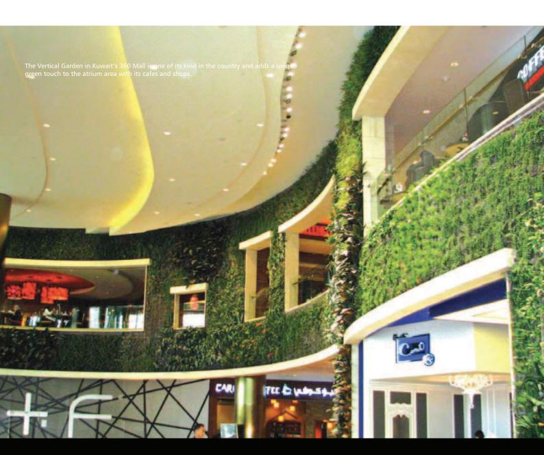
A one-centimetre PVC sheet is riveted to the metal frame and provides stability and waterproofing. The felt layer is stapled on the PVC. This layer allows an equal and homogenous distribution of water, which is always from the top (to imitate rainwater). The roots grow on and inside this felt. Plants can be introduced either as seeds, cuttings or grown plants.
